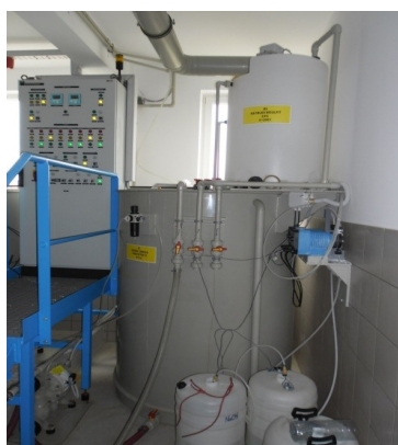
(a) Concentrate batch processing tank.
