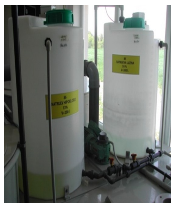
(b) NaOCl and NaOH dosing container.
